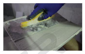
The adhesive should be spread in a straight line parallel to the short side of the ceramic tile to reduce the distance traveled by air being pushed out and obtain better adhesion.
