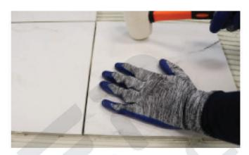
The adhesion coverage on the back of the ceramic tile should be as high as possible. Pressing the ceramic tiles on the substrate and break the adhesive ribs is a very important stage in installation of porcelain ceramic tiles and neglecting that, will affect the quality and durability of the adhesion.
