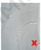
Place the porcelain ceramic tiles on the combed adhesive bed. For large size porcelain slabs, use runners and frames with suction cups. To break the ribs, move the ceramic tile at least the width of the ribs perpendicular to the ribs direction.
