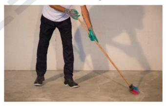
In order to reduce the surface water absorption and obtain better adhesion, it is recommended to apply primer. When installing porcelain ceramic tiles on absorbent substrates or in conditions such as direct sunlight and wind and also installing porcelain ceramic tiles in hot seasons, it is recommended to apply primer in two layers perpendicular to each other.
