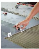
2- Then place the next ceramic tile on the other edge of the clip and adjust it by a rubber hammer.
