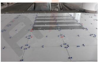
To ensure the leveling of the edges and avoid lippage between adjacent ceramic tiles, it's also recommended to use wedge and leveling clips.
