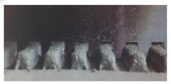
Using the hammer for applying pressure on the ceramic should be done in one step. After installation, even if a short time has elapsed (for example, 5-10 minutes), ceramic tile should not be tapped or pressed with the hammer. In such cases, it is recommended that the ceramic be removed from the surface and re-installed using fresh adhesive mortar
