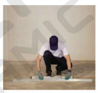
Then the substrate should be cleaned. The presence of dust, oil, etc. will have a negative effect on the adhesion of the coating on the substrate.
