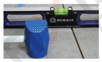
3- Place the wedge into the clip and fix it with the special pliers.
